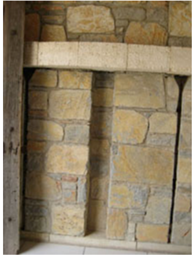
Figure 9. Stone wall detail at "The Marmara Bodrum" Hotel (photo credit: author)
